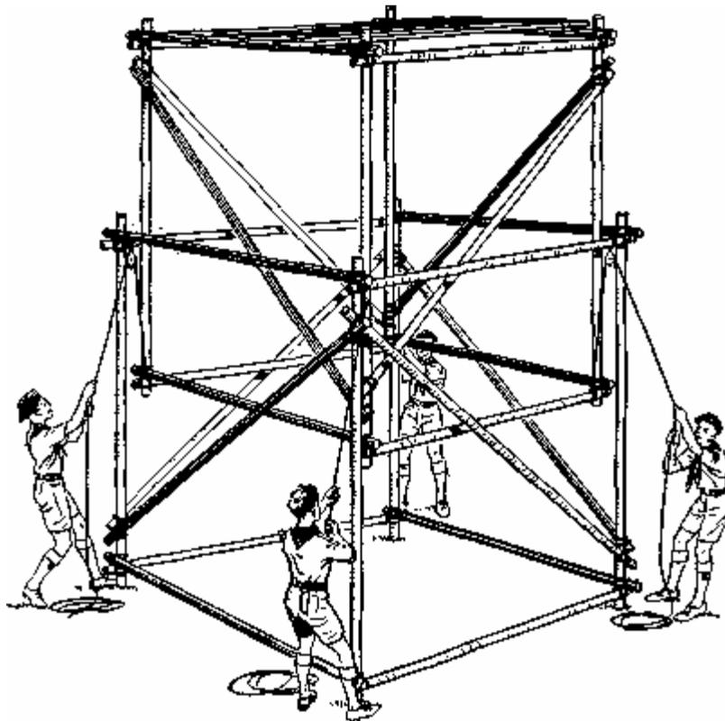
The Scouts who do the elevating must have a picket near by so that they can make fast when the inner tower has been raised to position.
